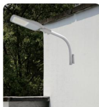
Wall bend installation
